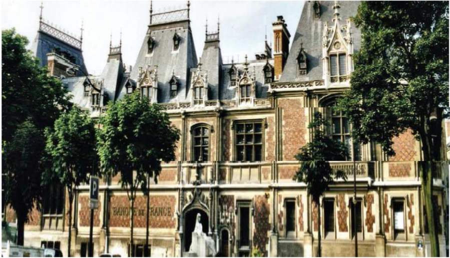
Façade and detail
